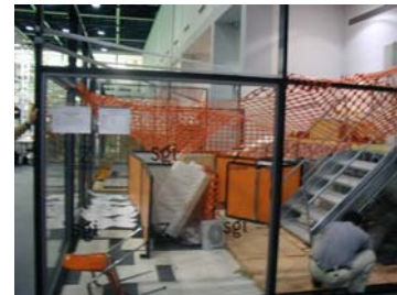
Figure 1: The Orange Arena
