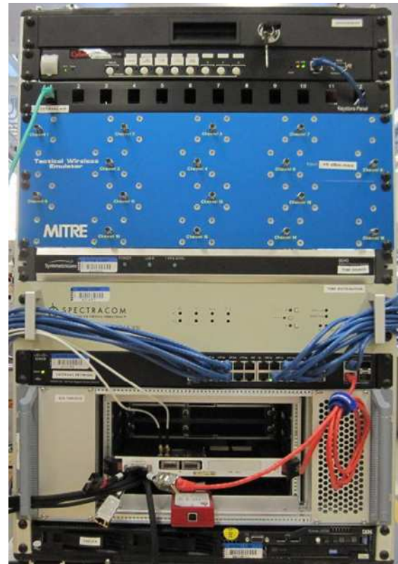
Figure 2. Front View of the TCES
